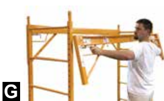
G Attach remaining Side Brace on opposite side.
