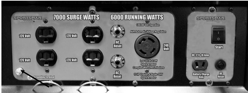
Figure 3 - Attaching the Grounding Wire to this Generator
