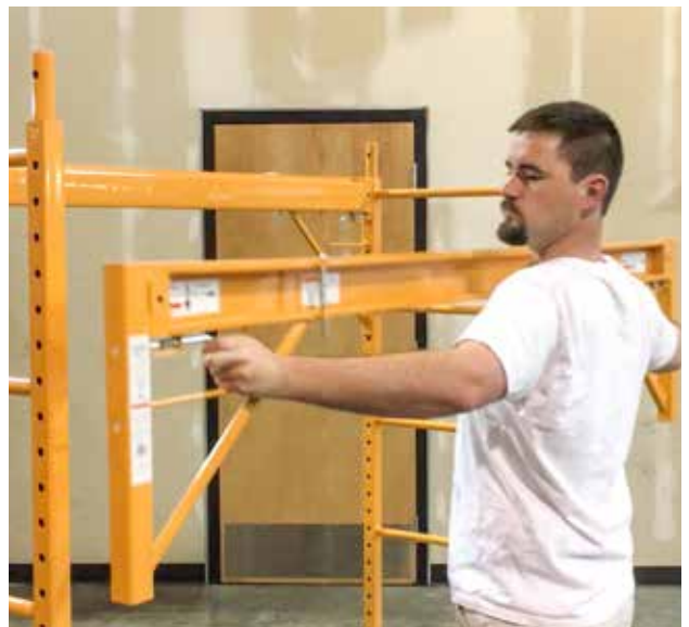
3 ATTACH SIDE BRACE
